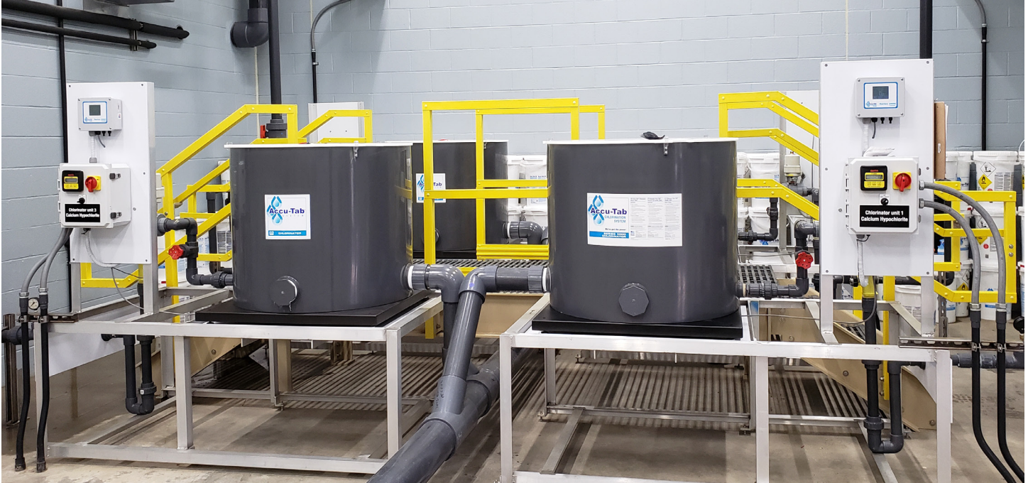
A bank of four Accu-Tab chlorination units at the Mon Valley Sewage Authority allow for a maximum of 400 lbs/hr chlorine delivery.
